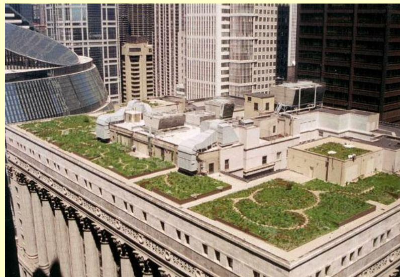
City Hall, Chicago, USA
