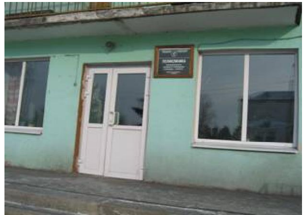
Replaced windows and doors in the hospital in Svirsk
